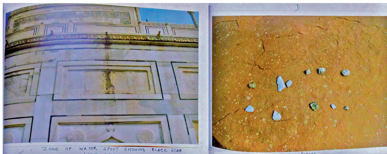
Fig. 1 Location of the samples investigated: water spout with and without black crusts (left side), pieces of crusts (right side)
