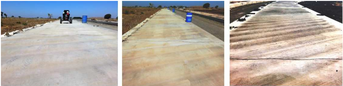
Figure 4.24: Low severity (left), medium severity (middle) and high severity (right) herringbone tracks respectively.
