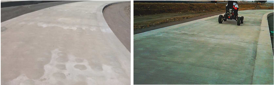
Figure 4.53: Left: rough road track. Right: Vehicle on rough road track.
