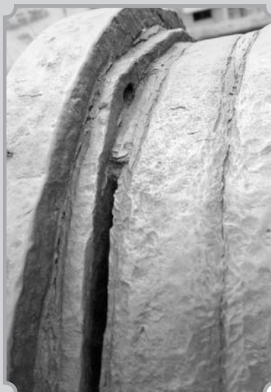
Figure A. A close-up view of one of the forge-welded joint regions on the outer surface showing that a smaller ring has been used to join the gaps between larger rings. The provision of a handling hole on the smaller ring should also be noted.
