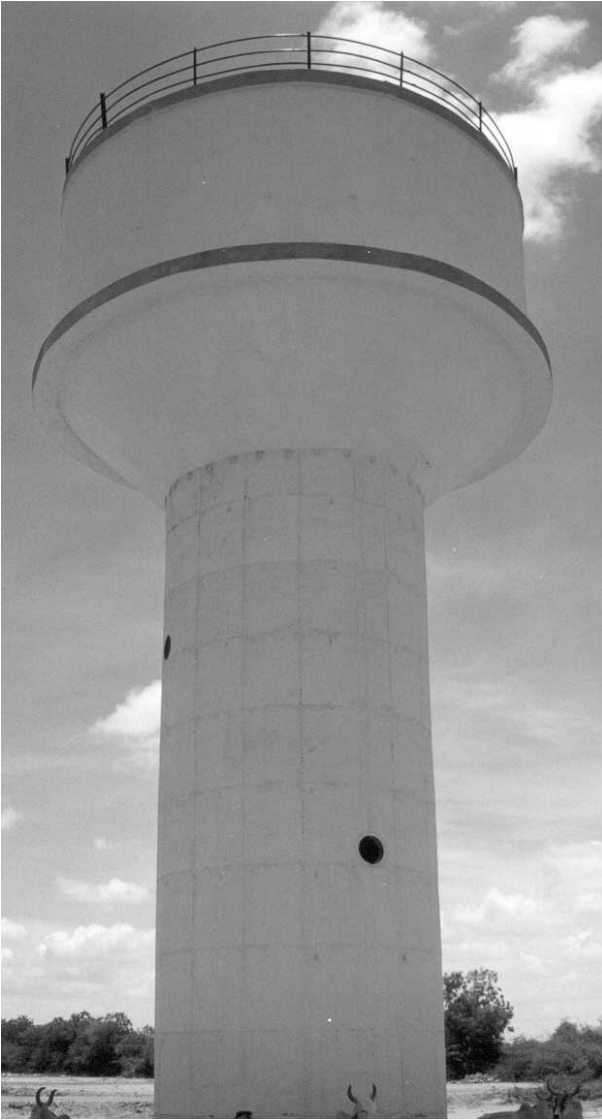
Figure 1. 200 kL Bhachau water tank which developed circumferential cracks up to one-third height of the staging. Severe cracking at the junctions of the first two 'lifts'.
