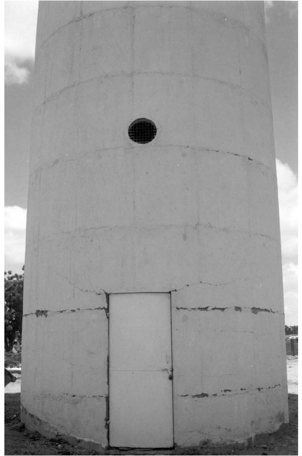
Figure 1. 200 kL Bhachau water tank which developed circumferential cracks up to one-third height of the staging. Severe cracking at the junctions of the first two 'lifts'.
