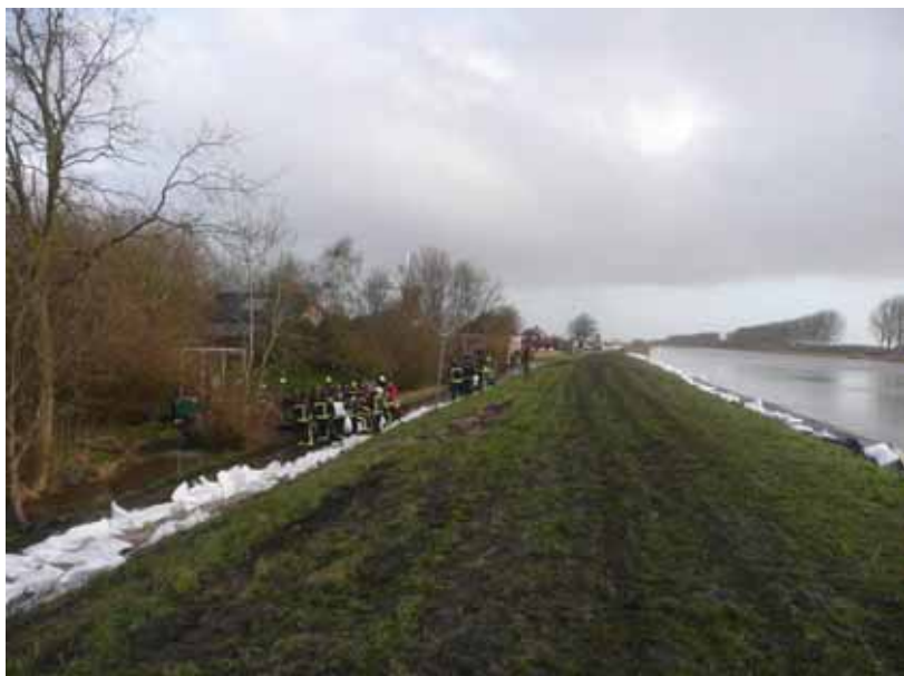
Figure 1. After the emergency, we remove the geosynthetics again and restore the levee into its original deplorable condition. Source Photo: Fugro
