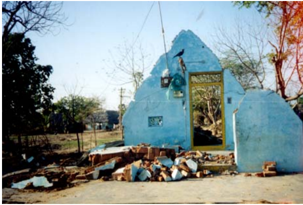
Fig. 7 A collapsed semi-engineered house at Muzukuthurai, near Pichvaram
