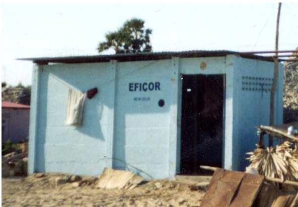
Fig. 11 A small-sized temporary shelter without adequate provision for light and ventilation
