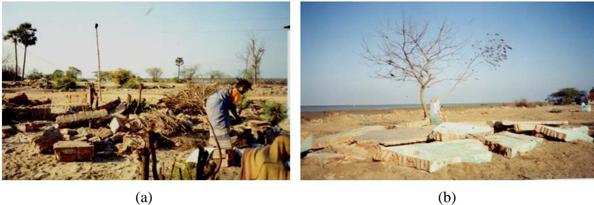
Fig. 6 (a) A totally ravaged hamlet in Cuddalore, Tamil Nadu, (b) Total collapse of a semi-engineered house in Muzhukuthurai, Tamil Nadu
