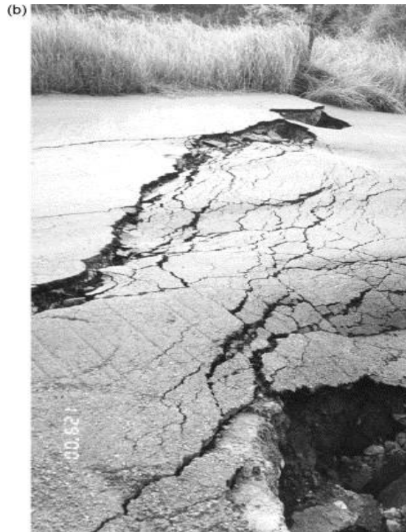
Figure 19: Nai Lu housing development site: (a) stable geo-synthetic-reinforced slope with vegetated facing, (b) severely cracked pavement along the road to the slope
