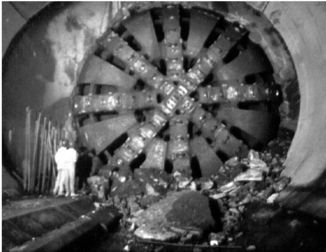
Athens Metro – 9.5m dia. open TBM
