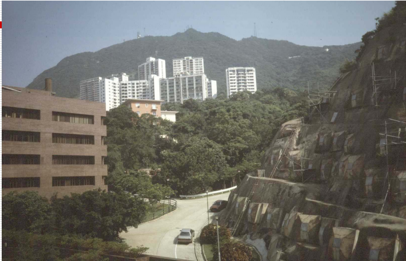
Remedial Measures for Unstable Rock Slope
