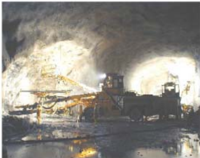
Computerised 3-boom drilling jumbos used in Singapore UAF caverns
