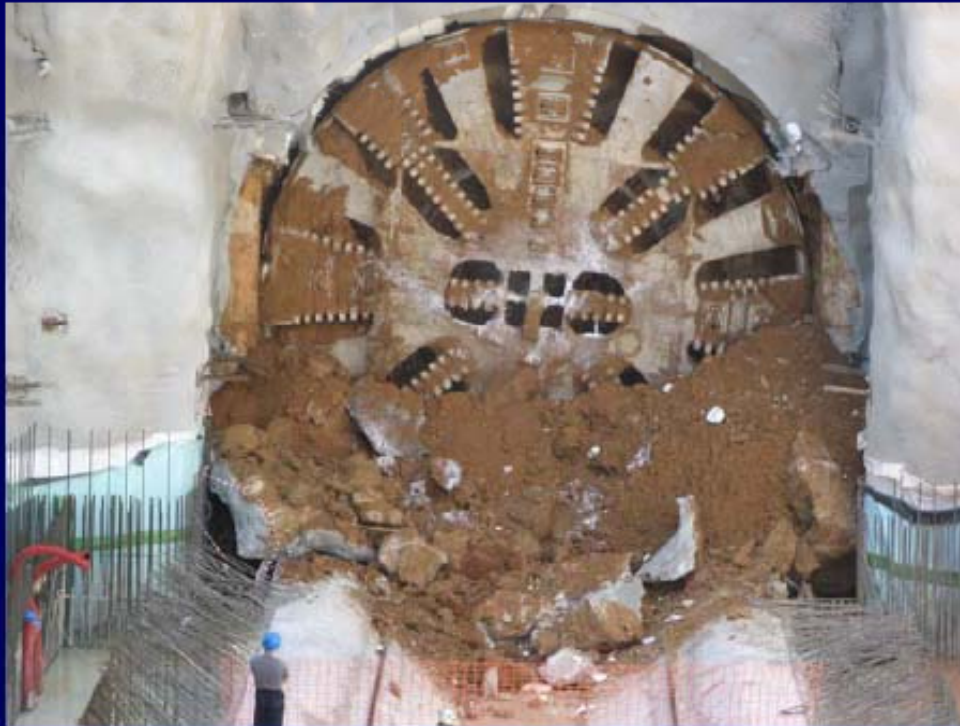
Elliniko station breakthrough
