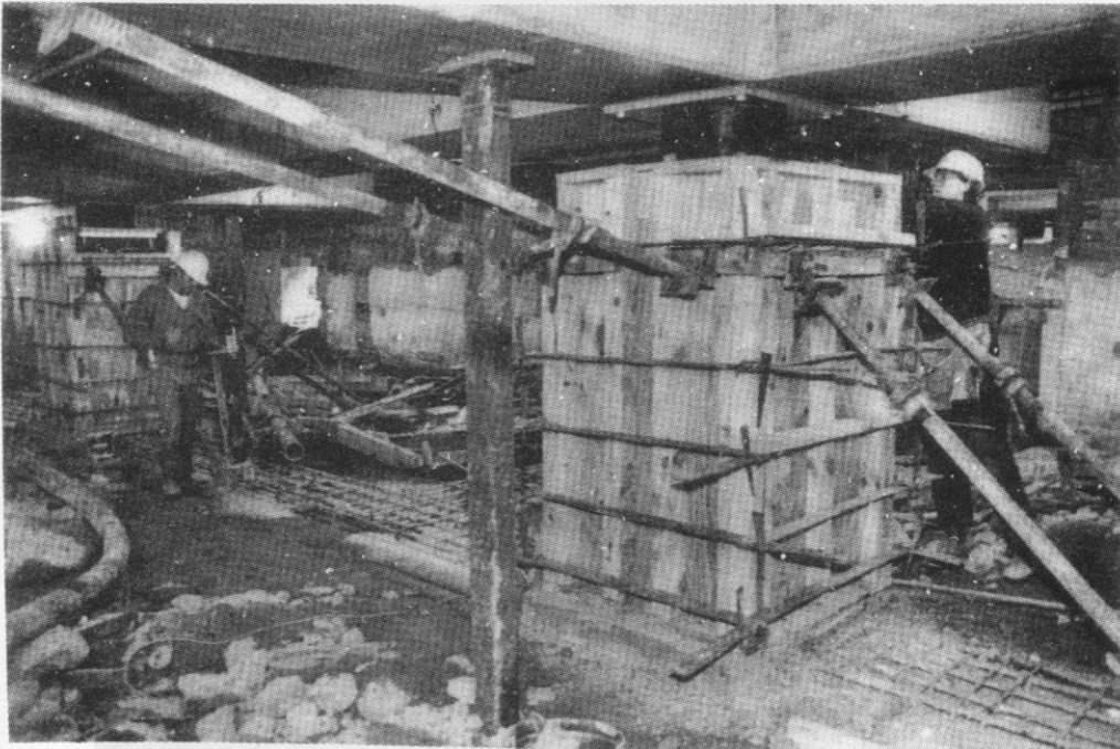
Fig. 12 Lead-rubber bearings being retrofitted under New Zealand Parliament
