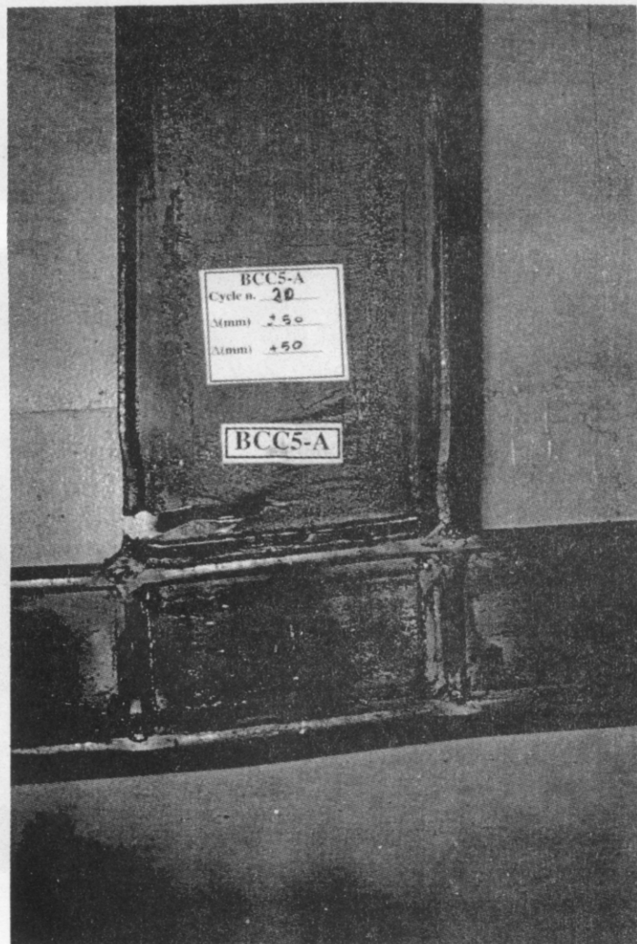
Fig. 14 Failure mode of a fully welded connection (BCC5)
