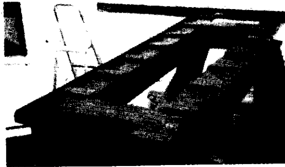
Fig. 7 Sliding bearings
