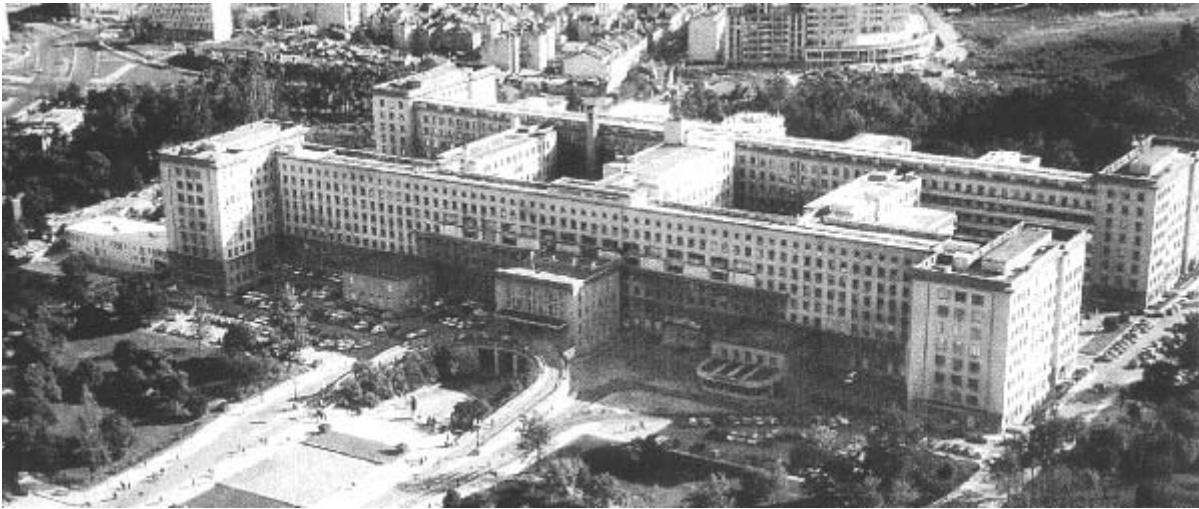
Fig. 1 Aerial view of the Santa Maria Hospital campus
