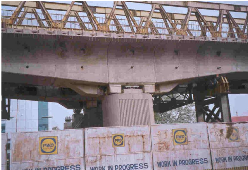
Fig. 6 Britannia Chowk Flyover: Elevation of restrained pier
