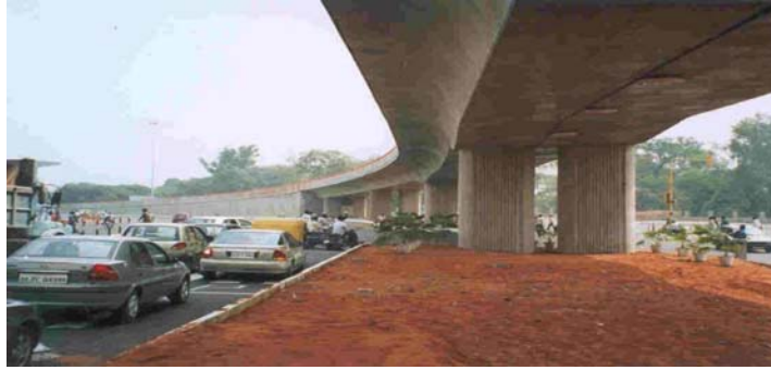
Fig. 11 Kalkaiji Flyover: Integral construction, high durability, low maintenance, increased safety during earthquakes
