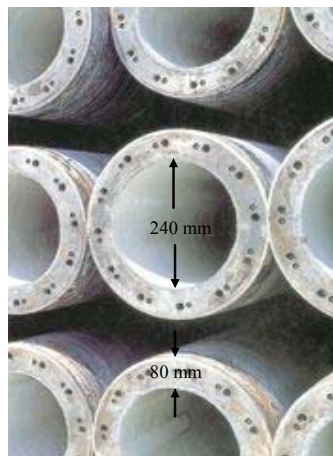
Fig. 7 Piles used in the building
