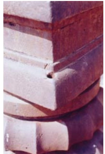
Figure 12. Holes in the lower base of the box pedestal.
