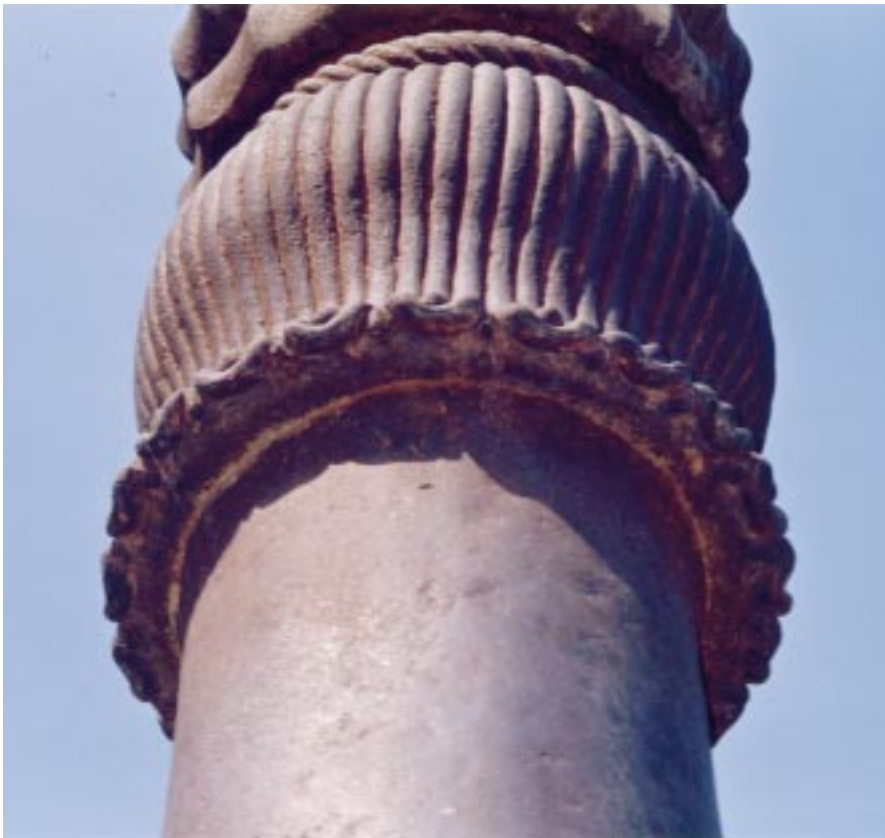
Figure 7. A bottom view of the joint between the pillar main body and the reeded bell section's base. Notice the nature of the rods that have been welded to the base.
