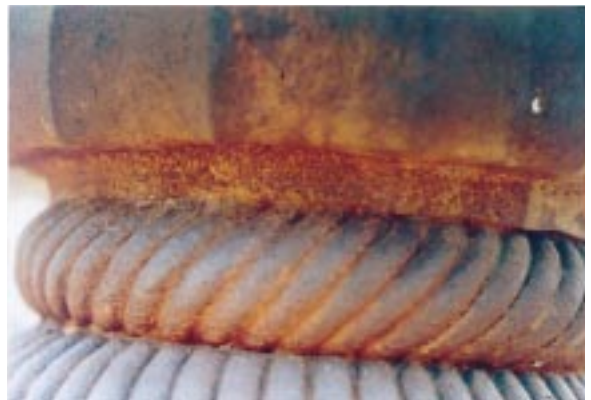
Figure 8. Details of the reeded slanted rod section of the Delhi iron pillar.
