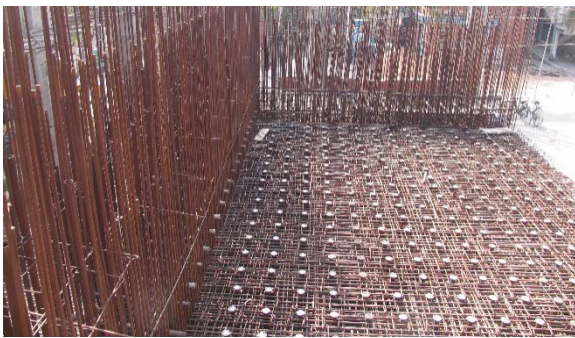
Mar 2009 Reinforcement of Strong Floor
