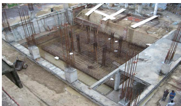
Nov 2007 Construction of Basement Walls
