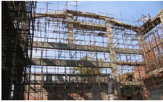
Mar 2009 Reinforcement of Strong Floor
