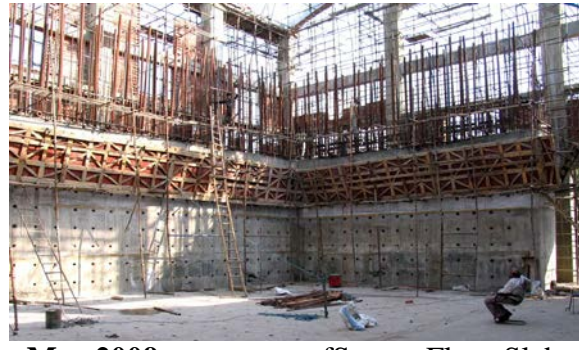
Mar 2009 Concreting of Strong Floor Slab
