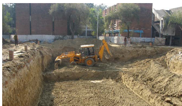
Dec 2006 Digging for the basement & foundn
