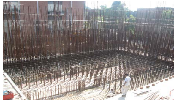
Oct 2008 Fixing of anchors' sleeves
