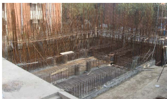
Nov 2007 Reinforcement of Reaction Wall & Basement
