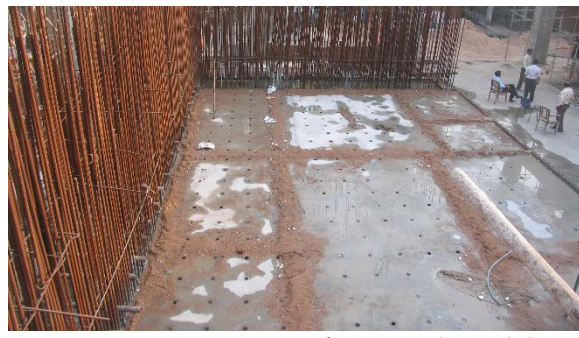
Mar 2009 Concreting of Strong Floor Slab
