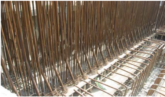
May 2008 Sheaths for post-tensioned walls
