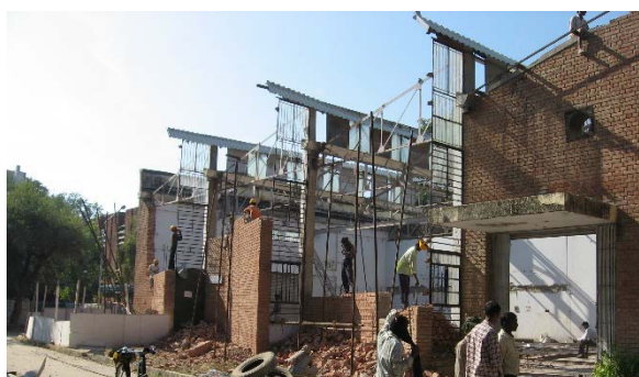
Nov 2006 Dismantling a part of existing Lab
