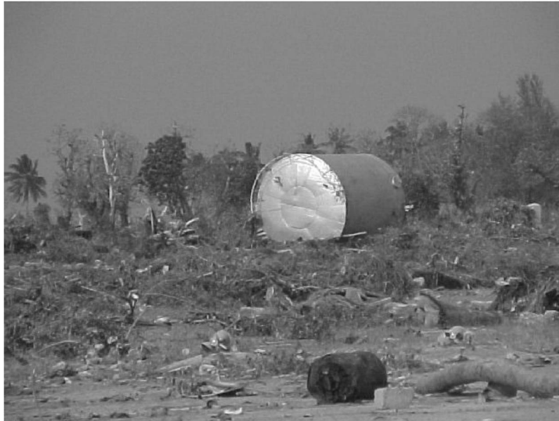
Figure 5. An oil tank of an electric power generator unit at the Air Force Colony in Car Nicobar Island was displaced by about 2 km to the end of the military airport runway (photo: S. Dash).
