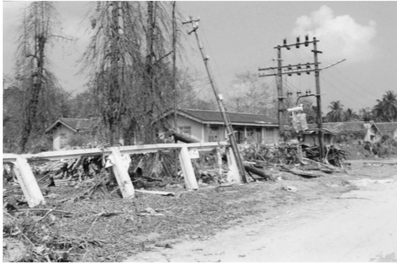
Figure 1. General wreck of the power distribution system at Hut Bay in Little Andaman Island (photo: S. Dash).
