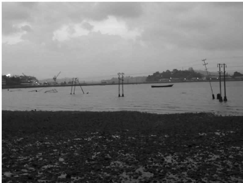
Figure 2. High-pressure tsunami waves damaged electrical poles near Haddo Wharf in Port Blair in South Andaman Island (photo: S. Jain).
