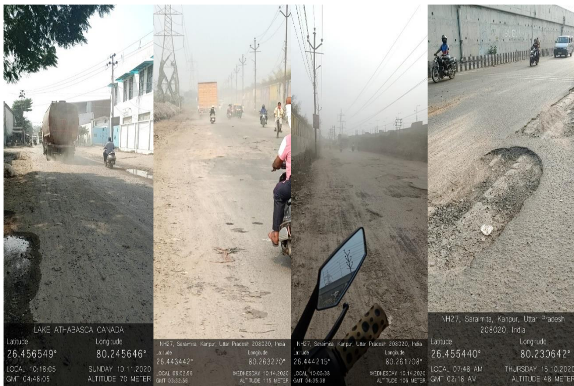
Figure 3.100: Broken roads causing higher road dust emissions
