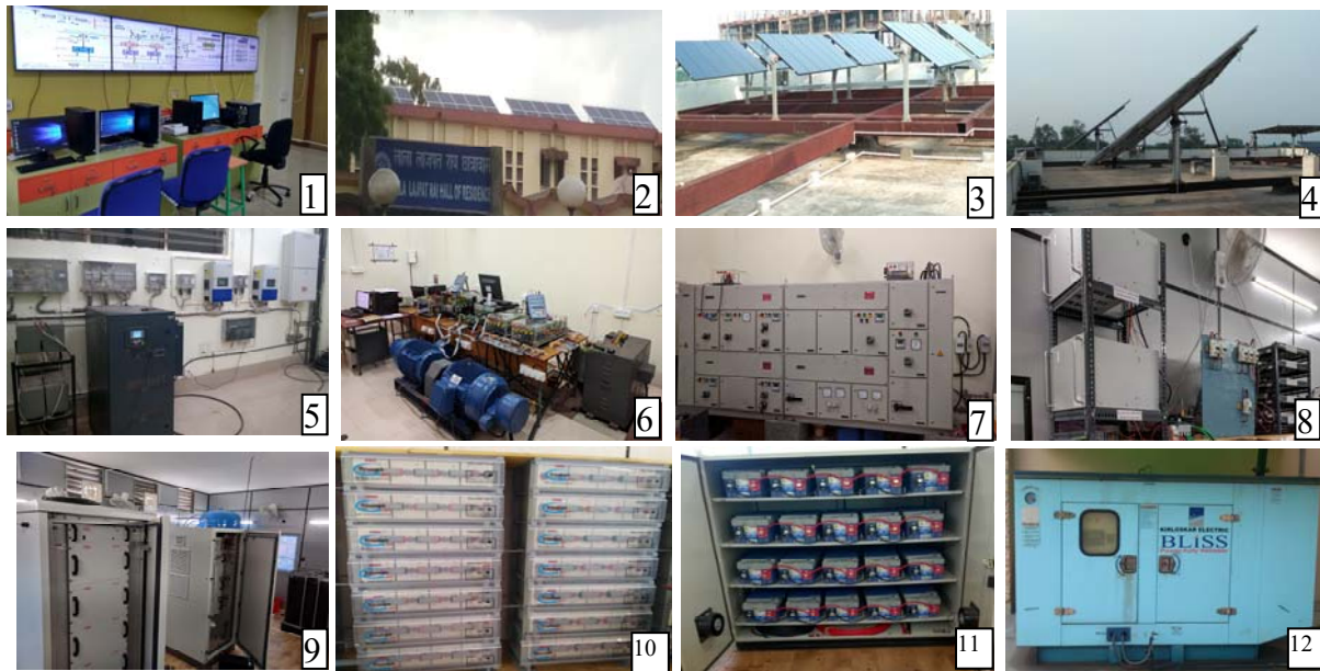
Fig.2: Photo of 1)Control Center, 2)100kW PV plant, 3)ThinFilm PV array with Single axis tracker, 4) Crystalline PV array with Dual axis tracker, 5) Hybrid and Grid-tied PV inverters, 6) Wind turbine-emulator & generator system, 7) HMG Interface panel, 8) Converters for Battery, SC and FC, 9)FC system with Electrolyser and H 2 tank, 10)Battery Bank, 11) SC bank, 12) Diesel generator
