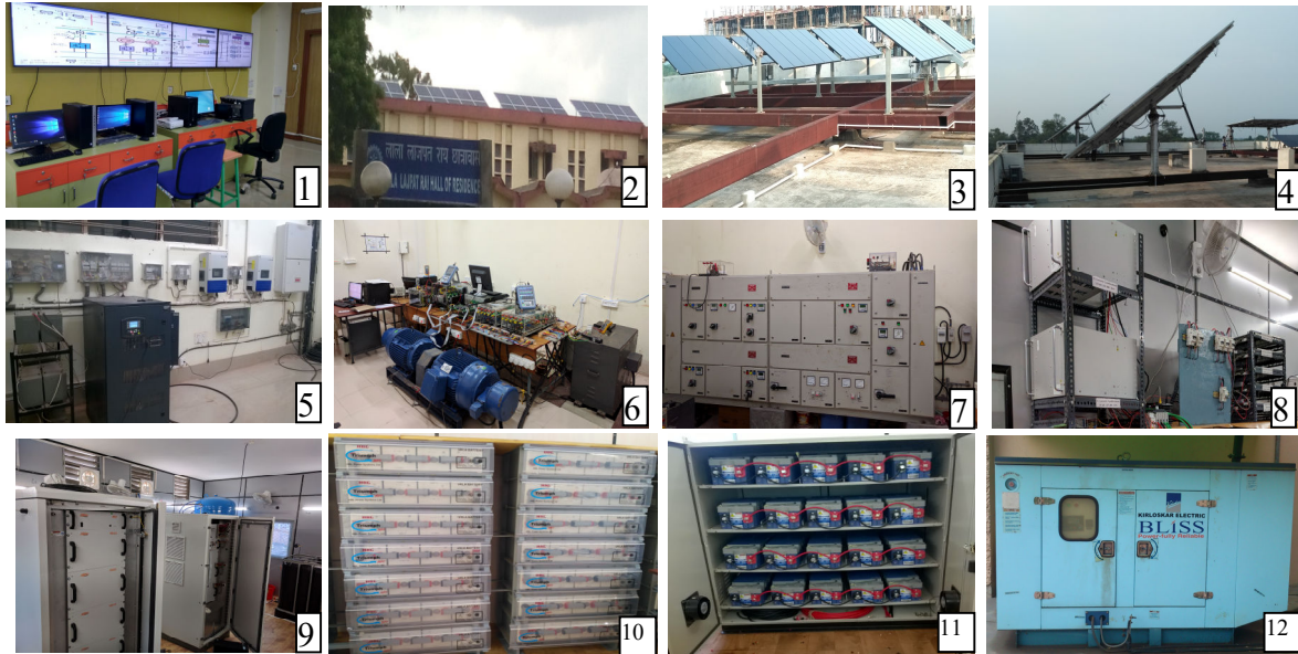
Fig.2: Photo of 1)Control Center, 2)100kW PV plant, 3)ThinFilm PV array with Single axis tracker, 4) Crystalline PV array with Dual axis tracker, 5) Hybrid and Grid-tied PV inverters, 6) Wind turbine-emulator & generator system, 7) HMG Interface panel, 8) Converters for Battery, SC and FC, 9)FC system with Electolyser and H2 tank, 10)Battery Bank, 11) SC bank, 12) Diesel generator
